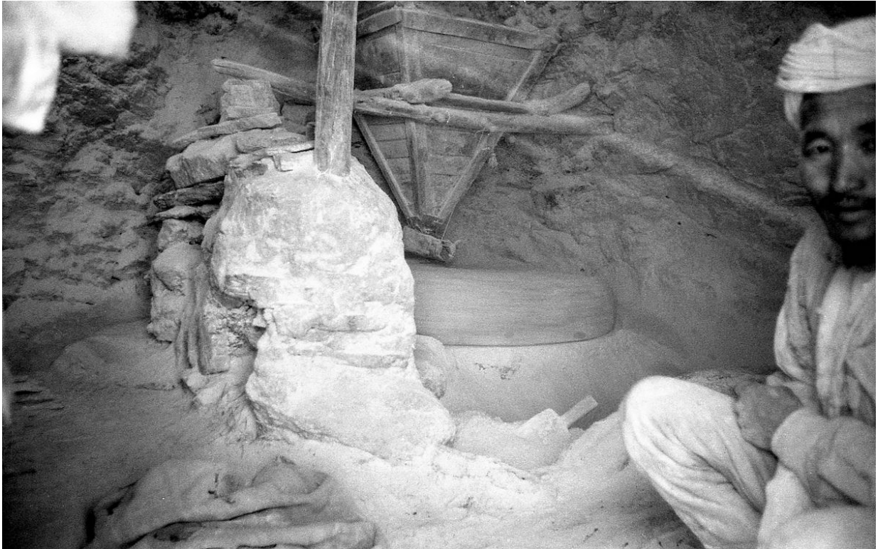
Inside: Gravity-fed, water-driven milling stones
